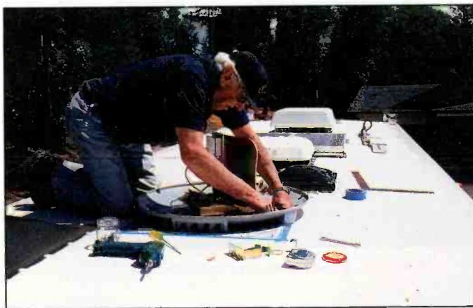
This silicone is just inside of the blue masking tape.
