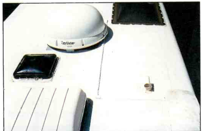
Feed the wires under the PVC and glue the PVC as you go. Try not to get the PVC cement on the wires underneath.
