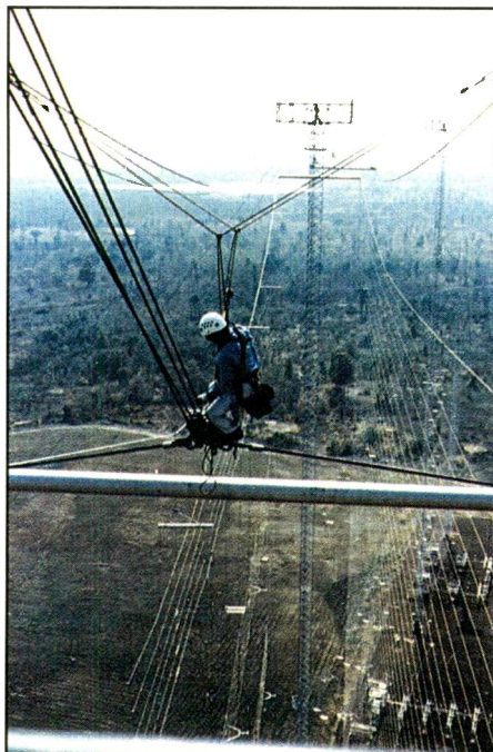
This VOA QSL showing work being done on an antenna system confirmed George Glotzbach's reception of RFE/RL!
