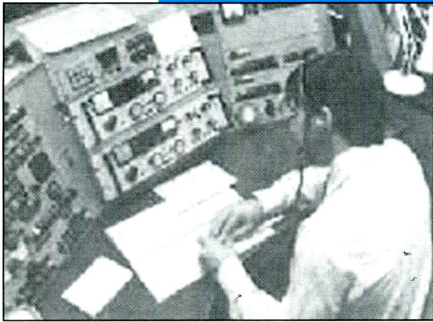
A view of contemporary operations. Notice the modular approach with redundancy in having multiple Eddystone EC958 receivers. Not shown are the AJAX brand transmitters housed in a separate room
