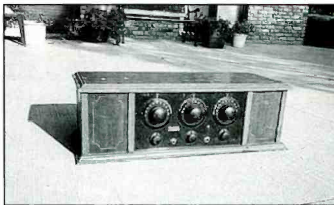
Here's Larry Shaunce's Lansing model M three-dialer TRF set from 1925.
