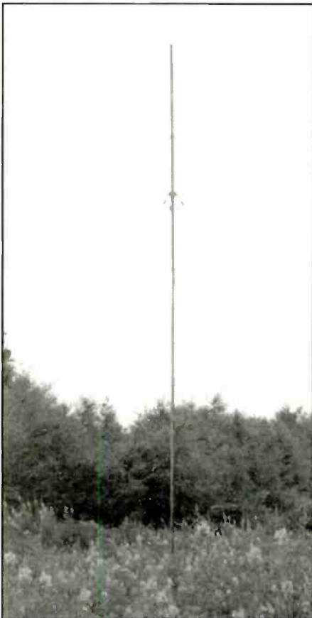
This antenna belongs to Canadian shortwave station CKFX in Vancouver, BC.
