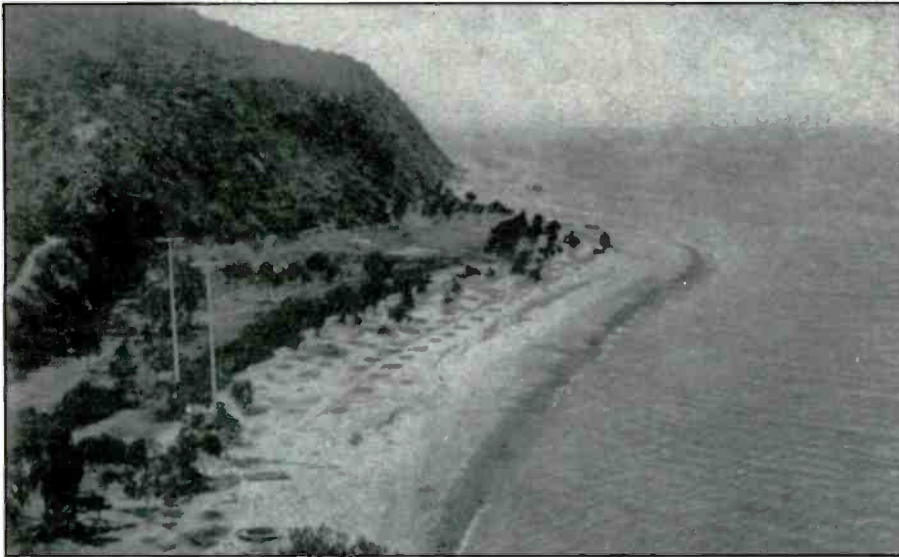
An early 1921 view of the site of Pacific Tel. & Tel. Station KUVX at Pebbly Beach, one mile from Avalon, Santa Catalina Island. This station exchanged telegraph and radiotelephone traffic with PT&T station KUXT on the mainland.
