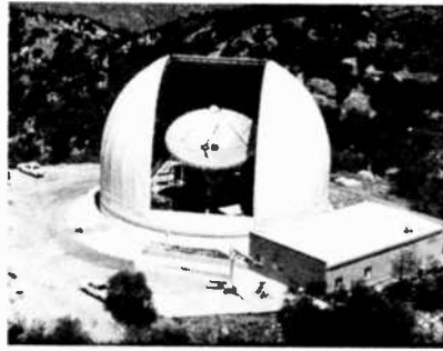
Some telescopes, such as those for the millimeter-wave region, are studying ultra-short-wave parts of the spectrum for the first time. One of those telescopes is the 36-foot millimeter-wave radio telescope at the Kitt Peak National Observatory near Tucson, Arizona (Photo courtesy of NRAO/AUI).
