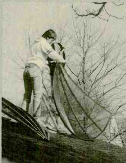
The first section is attached to the center hub with a single bolt.
