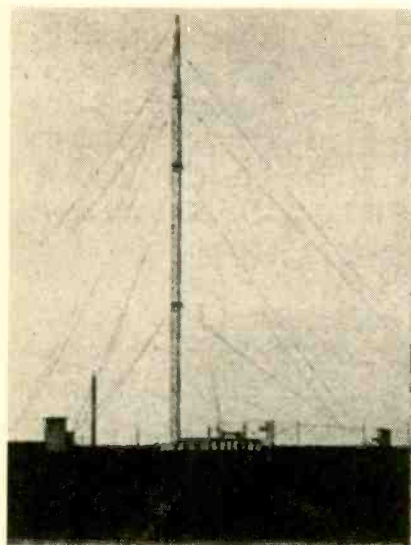
The main Sayville tower was the first in North America to substitute a ball-and-socket joint base for the more common "Eiffel Tower" design in which the structure supports itself. Most AM radio towers today use the Sayville design. The building at the base of the tower is the operations and transmitter building.
