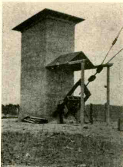
This large concrete and brick anchorage was one of six that supported the structure via thick cables. Note the large glass insulators.
