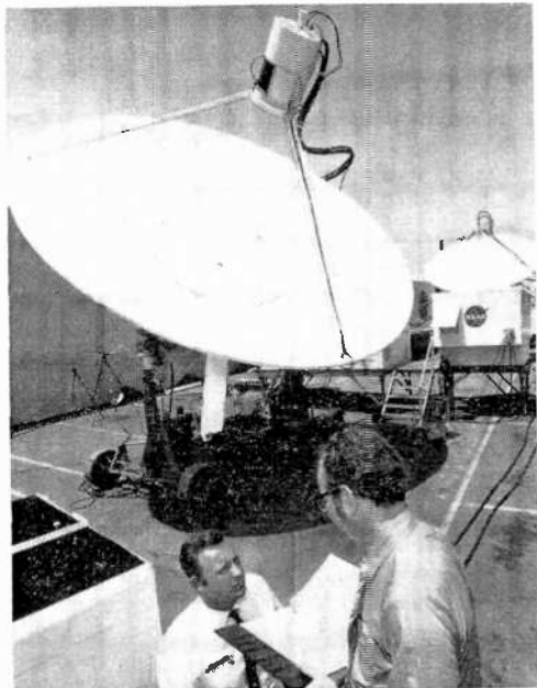
The new transportable earth terminal for satellites consists of a 21-foot dish (foreground) and a 15-foot dish with companion electronics in vans.
