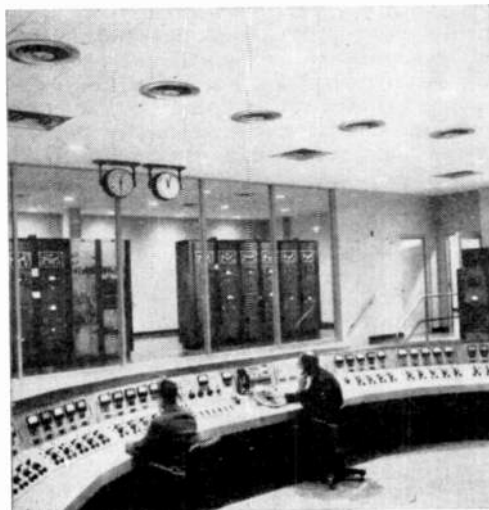
The Master Control Panel at the receiving station of the USIA's new broadcast complex at Greenville.
