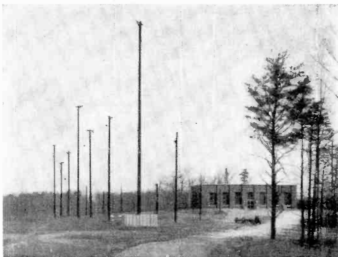
Some of the antennas used by Station WWV on its eight frequencies.
