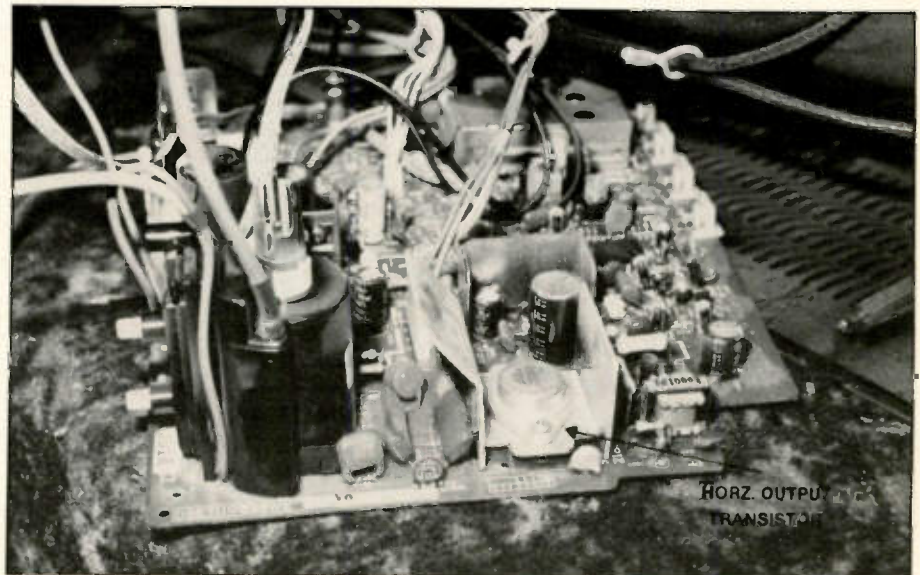
Figure 3. A leaky horizontal output transistor Q602 in one set caused the fuses to blow. Remove Q602 assembly with heat sink, by unsoldering board terminals.
