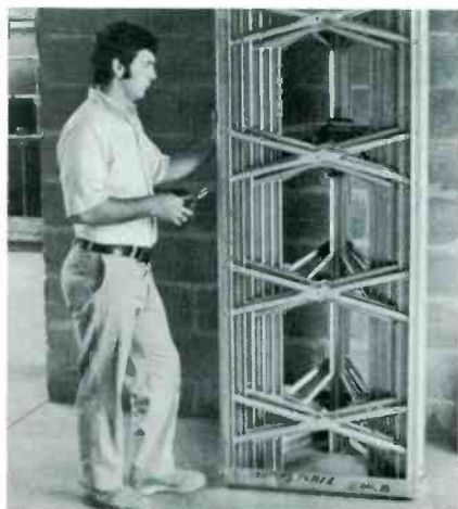
Step 1 Inspect the new tower when first received. Make certain it is the type you ordered, and that it is not damaged.
