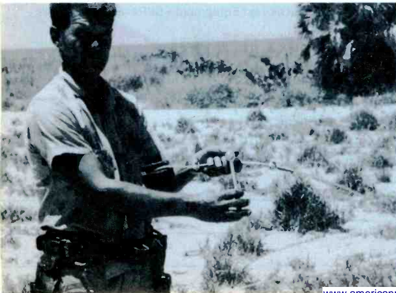
Tighten U-bolts on both sides of replacement strain insulator.
