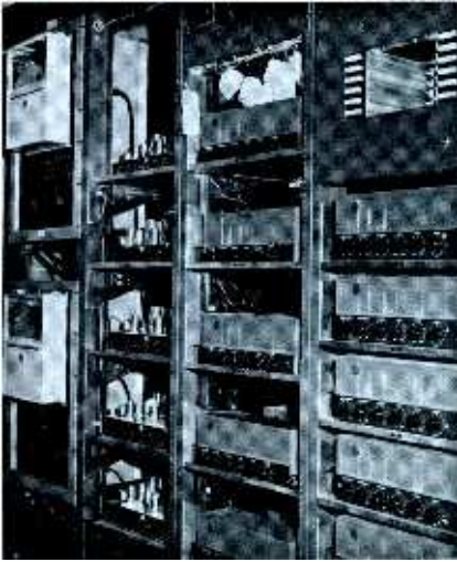
Fig. 13. Amplifiers and 14-track tape units.
