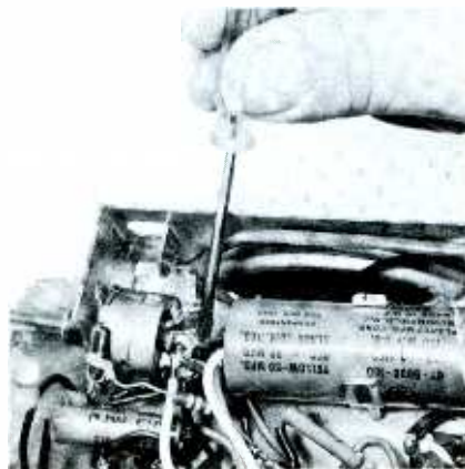
Fig. 1. Quick test for power switch.
