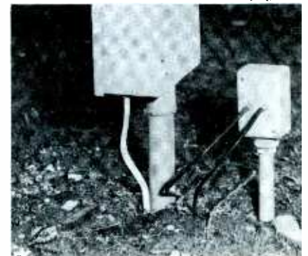
Fig. 3. Small outlet box is tap-off in a system that uses underground cable.
