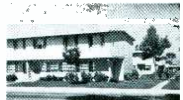
HOUSING PROJECT - 2,549 Wizards Installed To Date: L.A. Housing Authority, Los Angeles, California.
