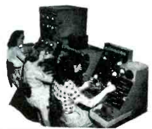
1ST FINISHED TUBE TEST All Raytheon tubes undergo a rigid 100% First Test where they must pass strict requirements on both physical and electrical characteristics. These girls are testing tubes for excessive noise and microphonics, inoperative tubes, specified electrical characteristics and physical appearance.
