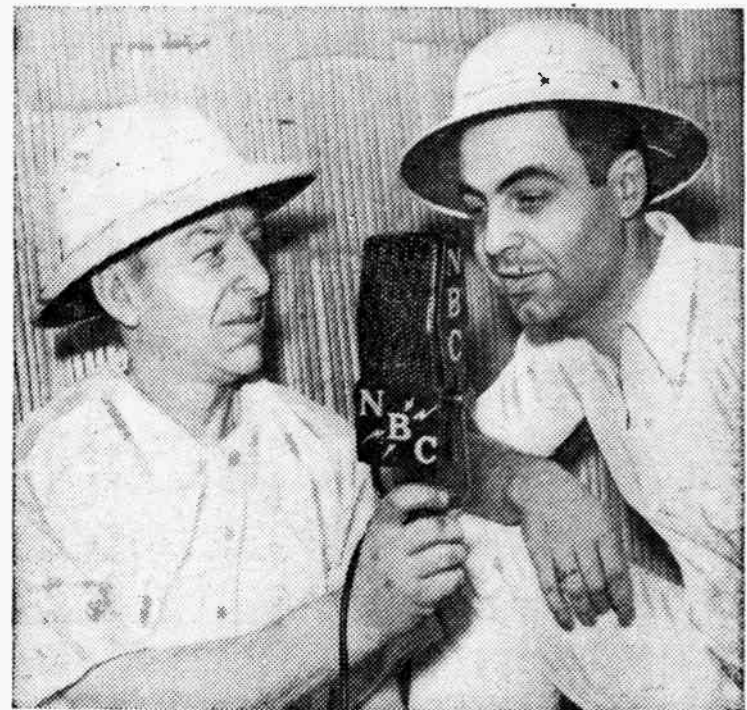
Erecting a new radio broadcasting station for the descendants of the mutineers of the H.M.S. Bounty on Pitcairn Island in the South Seas is a job entrusted to Granville P. Lindley (left) and L. S. Bellem, Jr. Broadcasts from the island are expected to be heard over NBC some time in March.
