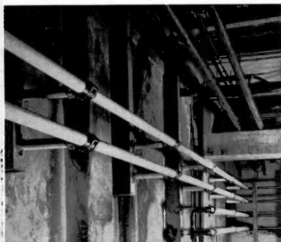
Straight line assembly of porcelain tubing in the water cooling system (bracing at end is temporary). Rollow Kimball, operator, shows how style-strip cover is removed from wiring duct under front of transmitter. The photograph at the right shows the compact and efficient water cooling system.
