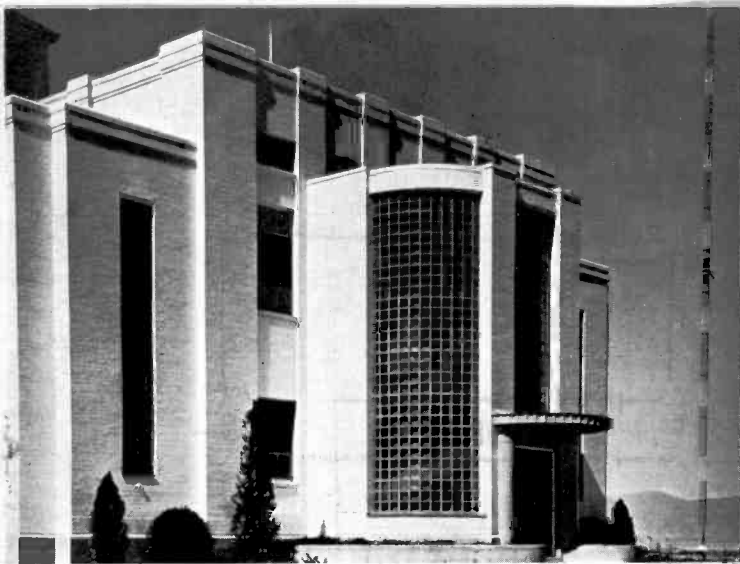
KSL transmitter building's new face and new 455 foot antenna. Circular structure at front encloses the new entrance stairway.
