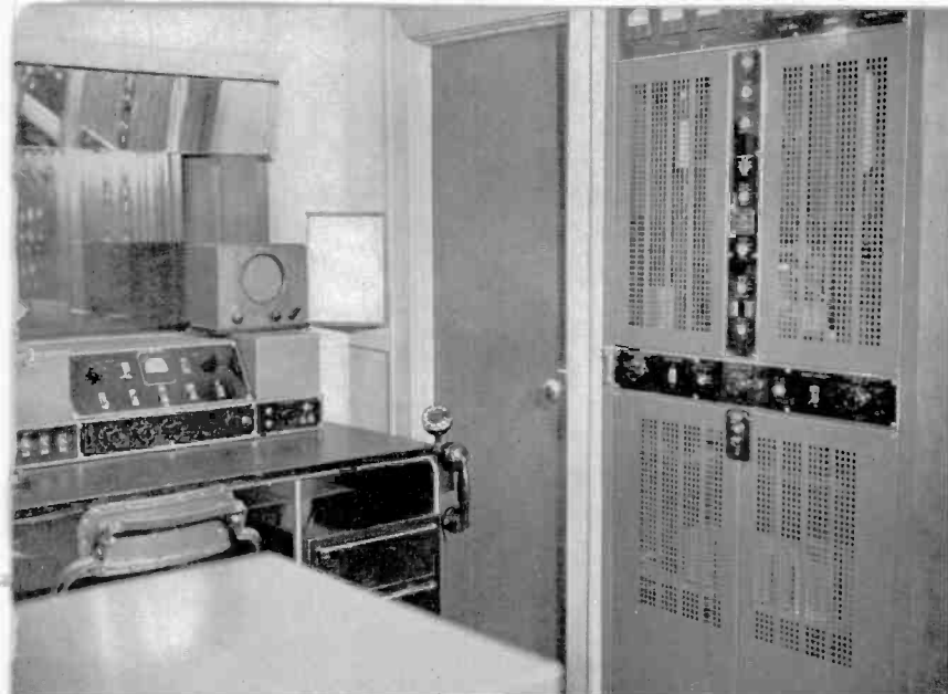
Above: The transmitter and control room, showing the 23B transmitter and, on the table, Western Electric 23A speech input equipment.
