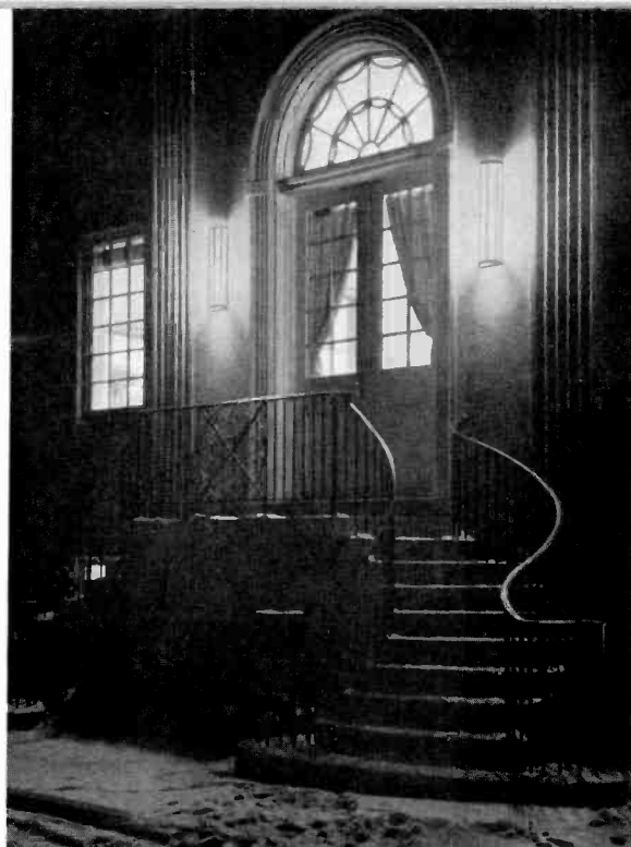
Behind these doors, the new Western Electric 50 KW.
