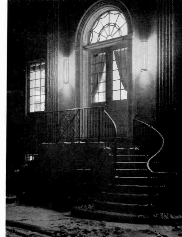
Behind these doors, the new Western Electric 50 KW.
