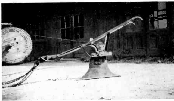
The "contraption" that was developed to lay-in the ground system. The reel is attached to the tractor that draws the plow.
