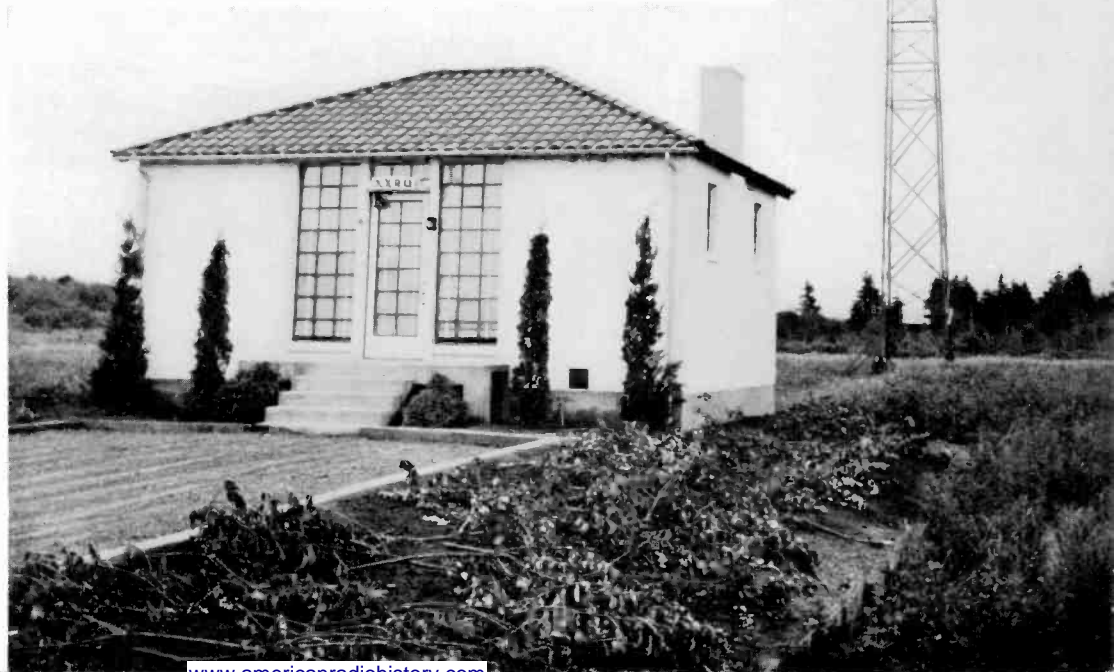
KXRO's modern transmitter building (right) which is constructed of concrete and stucco. The 189 foot Blaw-Knox radiator in background.
