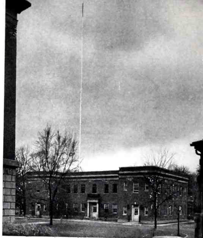
White Plains police headquarters where the heart of the Western Electric two-way police radio system is located. Because the coaxial type antenna is used, an unusually strong signal is obtained. Bottom panel: Radio equipped motor patrol fleet ready for action.
