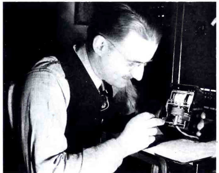
Clifton Todd, Chief Engineer, WNAX, showing his automatic temperature indicator.
