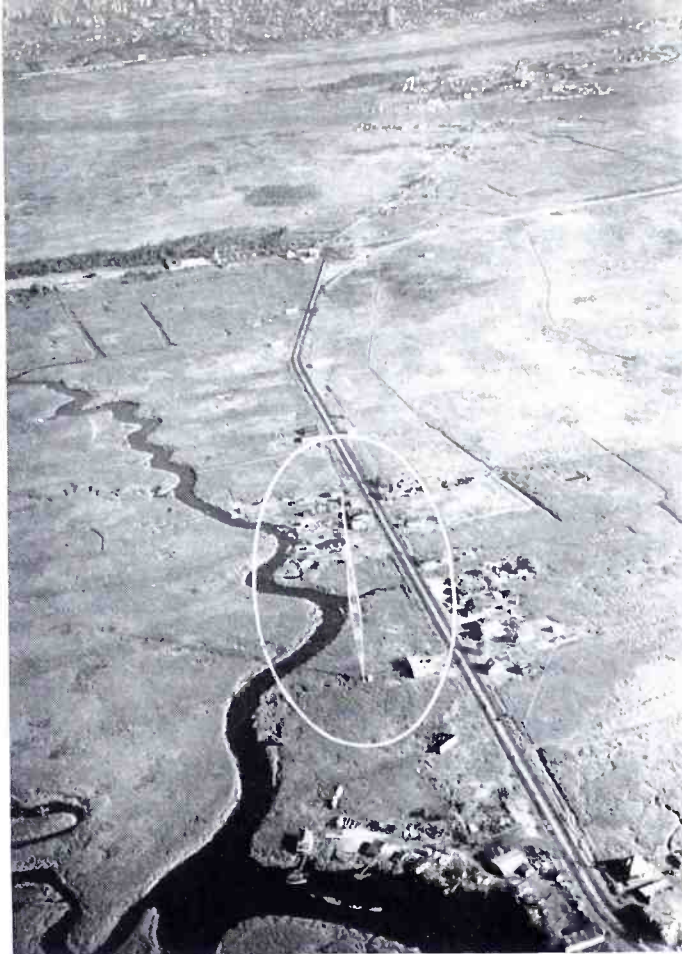
WNEW transmitter site at Carlstad, N. J. With tidal water lapping its antenna base, an almost perfect ground is obtained.
