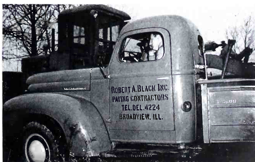
"Need six more loads of sand . . . fast!" For routine messages and in emergencies this Broadview, Ill., paving contractor finds the mobile telephone service provided by the Illinois Bell Telephone Company indispensable in his work.
