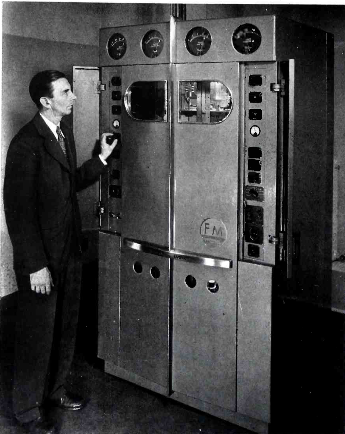
Above: Carson Donaldson, chief engineer, stands beside KUSC's Western Electric FM transmitter, operating on a frequency of 91.7 mc. Transmitter power is 1 kw, licensed effective radiated power is 2.9 kw.
