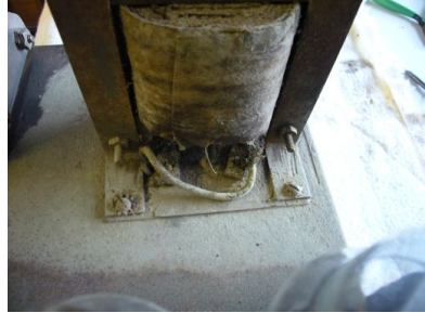
Power transformer with taps
