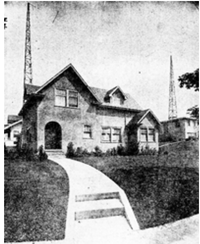
Original Portland home of KPOJ at 36th and Glenwood in Eastmoreland district. Transmitter and studios were both located on second floor of garage seen in rear.
