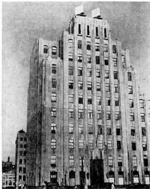
The Boston terminal of the Bell System radio relay route between New York and Boston is situated in the Bowdoin Square Building of the New England Telephone and Telegraph Company. The special microwave antennas which receive and beam the communications signal can be seen on the roof.
