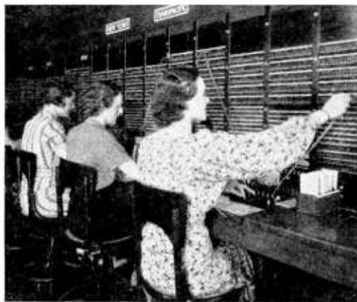
San Francisco. The switchboard through which Radio-telephone calls flow between shore and ships in the Pacific Ocean.
