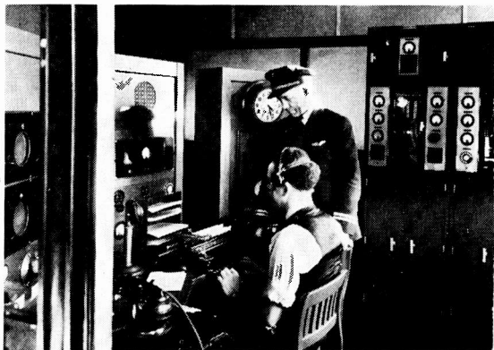
Ground Station of EAL at Newark Airport
