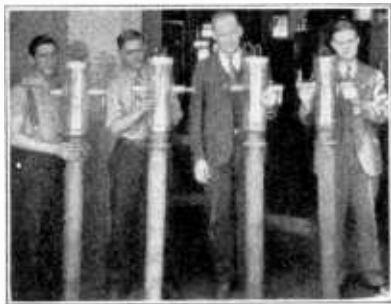
Four 100 kilowatt tubes outside their jackets.
