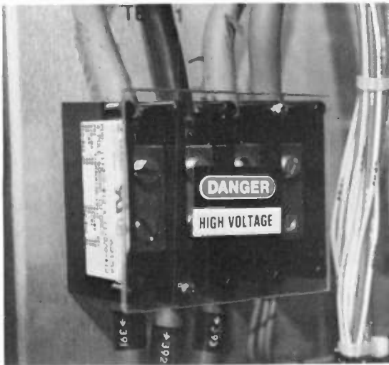
FIGURE 11. GUARD FOR AC TERMINAL BLOCK
