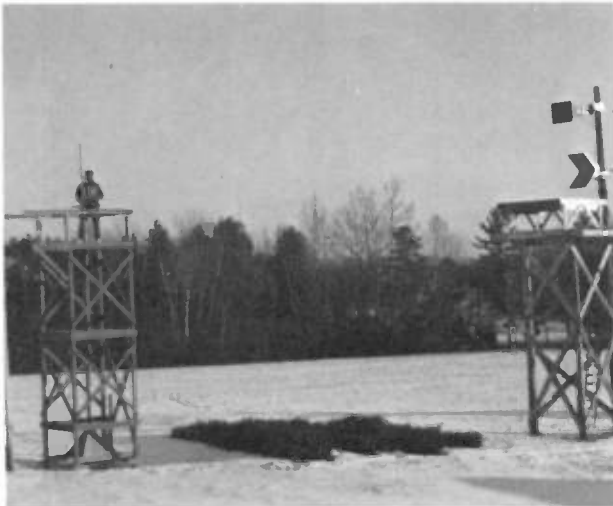
Figure 8 - Antenna manufacturer's test range. (courtesy Shiveley Labs)
