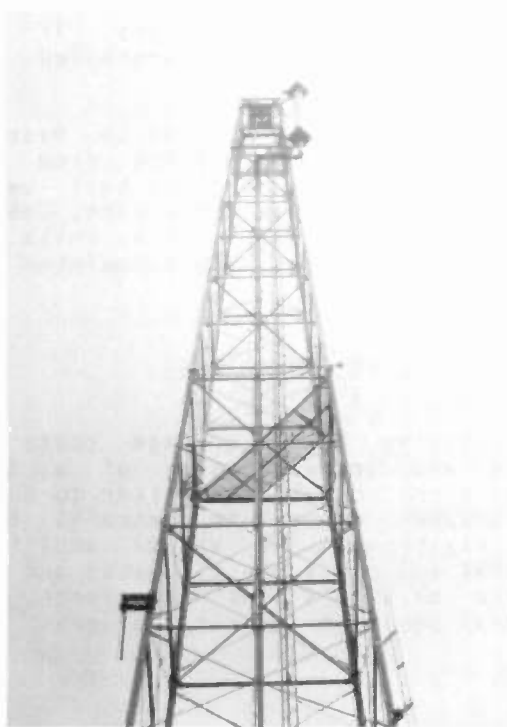
Small, side-mounted temporary antenna
