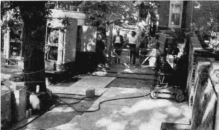
FIG. 5-29. A "Public Space" permit was required for this Person-to-Person remote because the sidewalk was needed for camera and Fearless dolly operation. The mobile unit occupied public space for approximately 12 hr and also required permit. Electric power was fed to distribution panel (see Figs. 5-30 and 5-31) from manhole in sidewalk.
