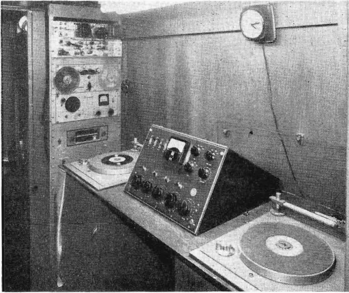
FIG. 4-7. Interior of vehicle, note rack-mounted equipment.
