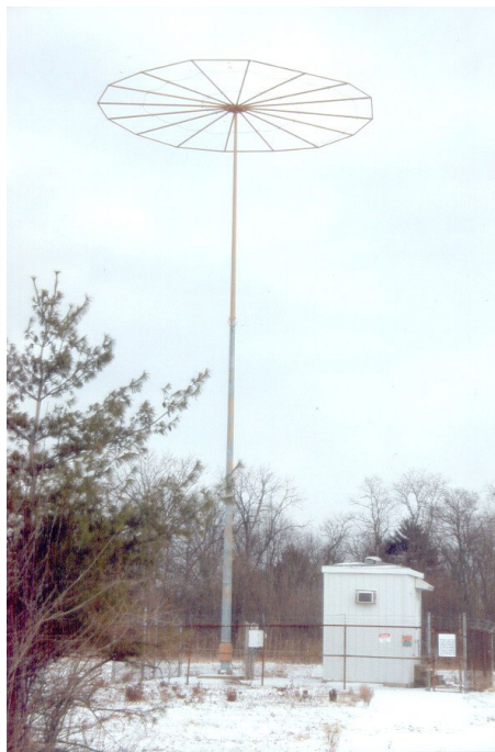
Unmanned, low power beacons like this one await your DXing skills. (MDE, 379 kHz, Cincinnati, OH)
