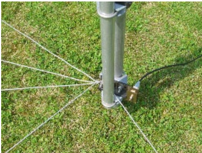
A somewhat modest system of ground radials for a vertical.
