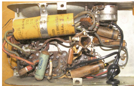
The Arvin's cramped chassis makes capacitor replacement an adventure.
