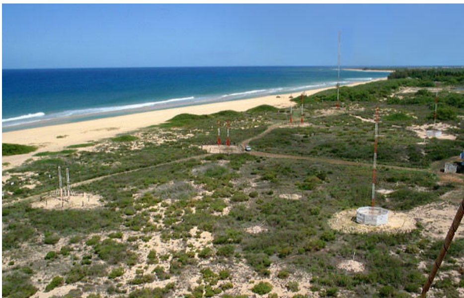
WWVH, Kauai, Hawaii antenna field. Left to right: 20.0 MHz array (abandoned), 15.0 MHz array, 10.0 MHz array, 2.5 MHz dipole, Standby 1 (SB1) broadband, and Standby 2 (SB2) broadband (Courtesy: NIST)
