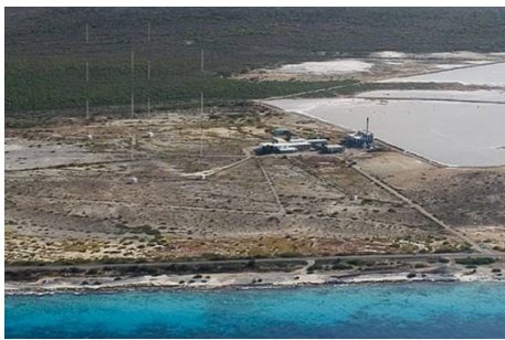
TWR-Bonaire is situated on the southwest coast, adjacent to a solar-salt company, giving it excellent ground conductivity.
