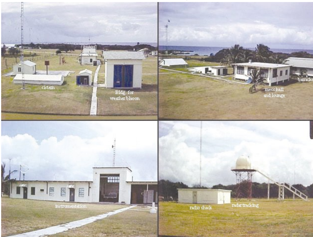
The National Weather Service compound in 1972 (Don Keith)
