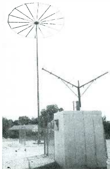
FIG. 2. Newer beacon sites often employ a vertical top hat antenna.
