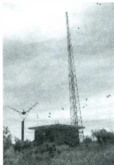
FIG. 3. "Hot tower" antennas are common at beacon sites and other LF utility stations
