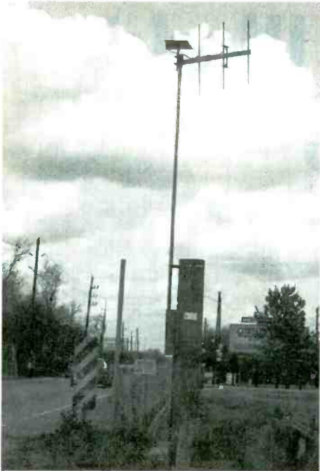
The frequency counter snagged this Yagi used by the flood control district transmitting at 169 MHz.
