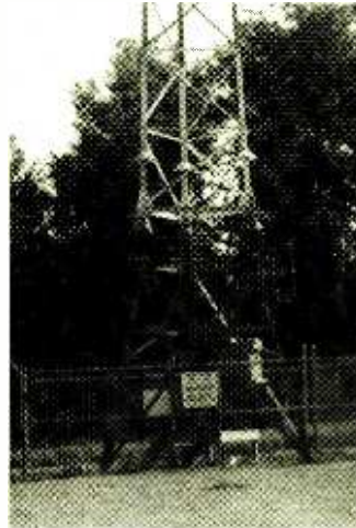
A close-up view of the tower base at beacon "O", 344 kHz in Ottawa, Ontario. The overall tower height is about 175 feet. (Photo submitted by Jacques d'Avignon, VE3VIA)
