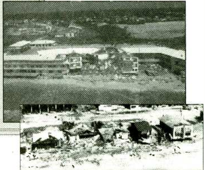
Beach damage from Hurricane Opal taken by Beau Hannah, courtesy of the U.S. Army Corps of Engineers.
