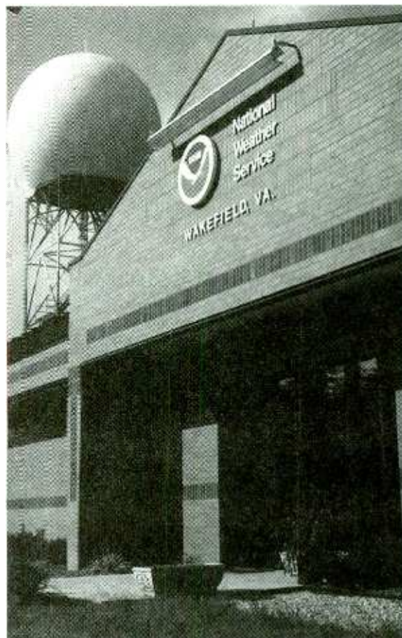
The pride of Wakefield, VA. Entrance to the new National Weather Service Office. Doppler NEXRAD radome in background.
