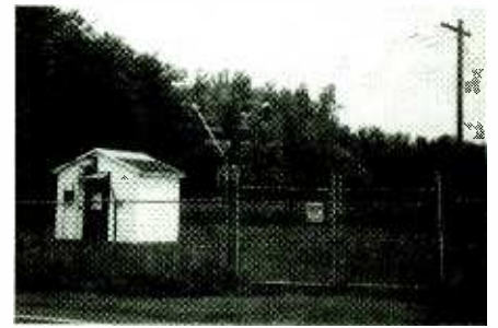
Beacon SY (242 kHz)—East Syracuse, NY (The V-shaped antenna beside the building is for a 75 MHz marker beacon.) Photo by Philip Gentile
