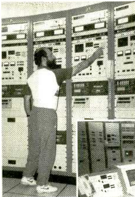
Left: Although the transmitters can be completely controlled by computer, the technicians must be prepared to manually select the time-on/time-off, frequency, appropriate antenna, antenna take-off angle, antenna slew angle, and program. Each of the ten 500-kW transmitters has a control rack. Four of the racks are shown here.
