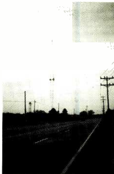
WLW-700kHz, Cincinnati, uses this impressive single tower near Mason, Ohio. Again, this single-tower system indicates that WLW is a non-directional station.
