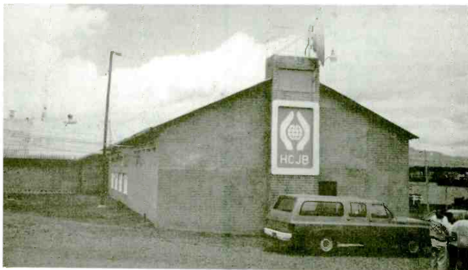
HCJB's transmitter building at Pifo, Ecuador.
