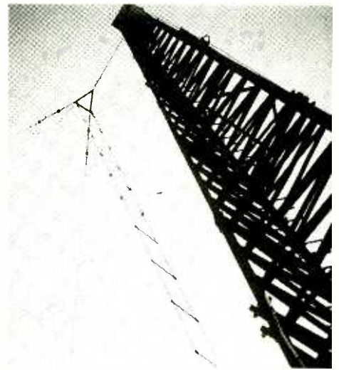
Eavesdropping at the pro’s: One pole of a large rhombic antenna.
