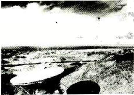
Ascension Island transmitter with dish.
