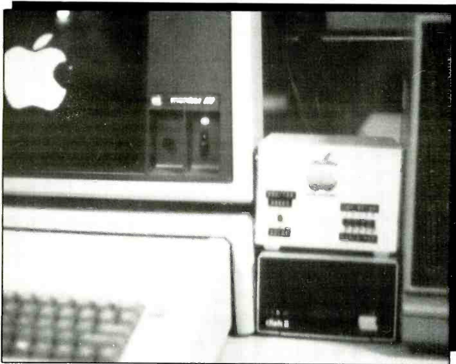
Fig. 2. Label all switches on the front panel for easy identification.
