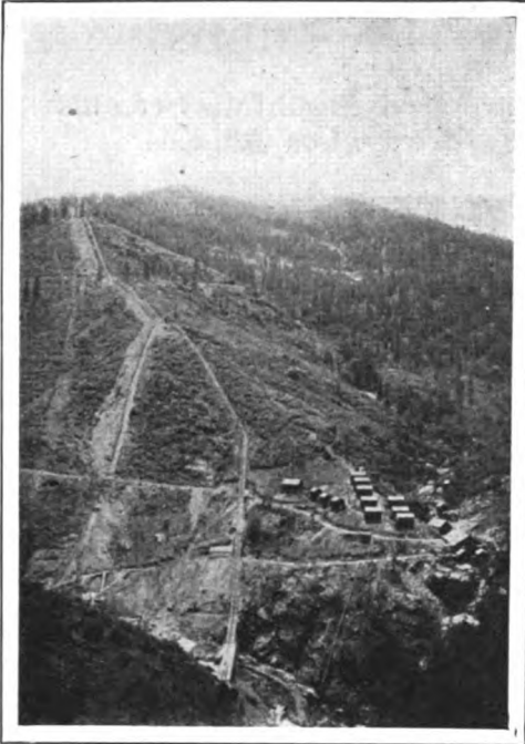
THE INCLINED RAILWAY AT POWER HOUSE NO. 2. THIS RAILWAY RISES FROM 3,800 TO 4,800 FEET AND HAS A TOTAL LENGTH OF 6,000 FEET. A GROUP OF SHACKS USED BY THE WORKMEN MAY BE SEEN AT THE RIGHT
