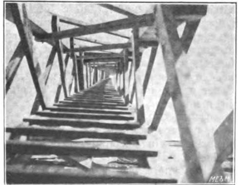
LOOKING UP THROUGH THE CENTER OF THE AERIAL MAST
