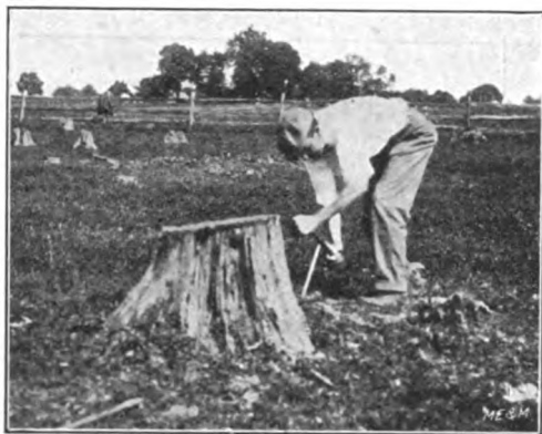
BORING A HOLE FOR BLASTING A TREE STUMP
