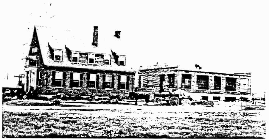
View from North of the facility. This building was to eventually have the rear wall knocked out to contain the 500 KW monster. This construction took place in 1928 to house the 1927 Western Electric 50 KW rig.
